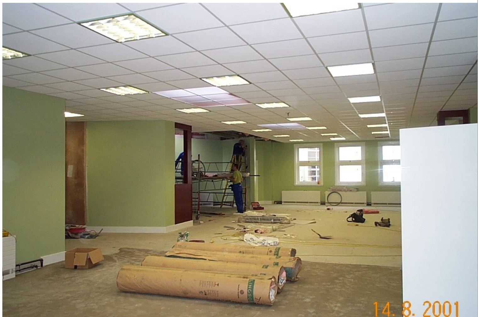
St. Bridget's@ Dining Hall under construction
