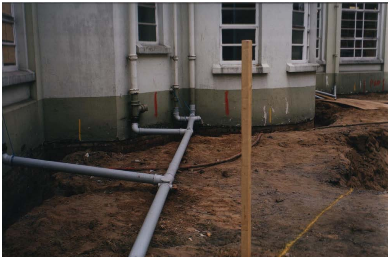
St Bridget's, Baillieston: Drainage diversion before foundation dig
