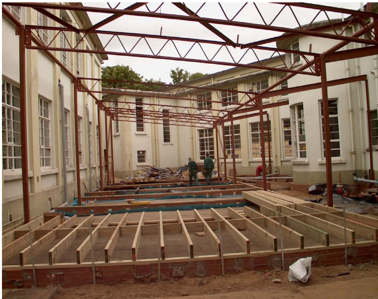
St Bridget's, Baillieston: under construction
