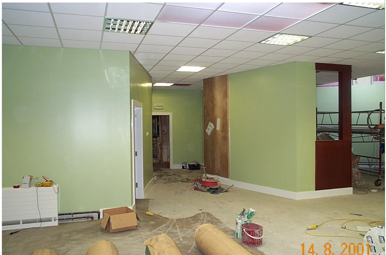
St. Bridget's: Dining Hall to main access
