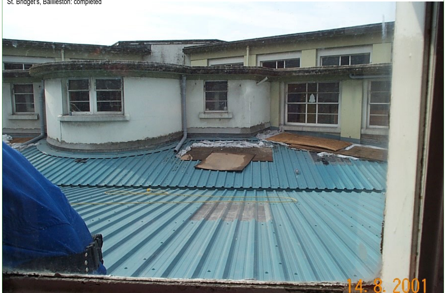
St. Bridget's: under construction
